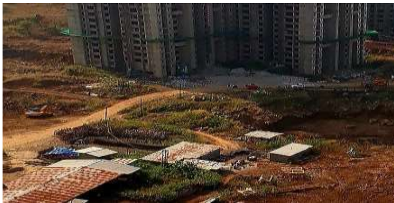
E 1 Building/E2 Building
